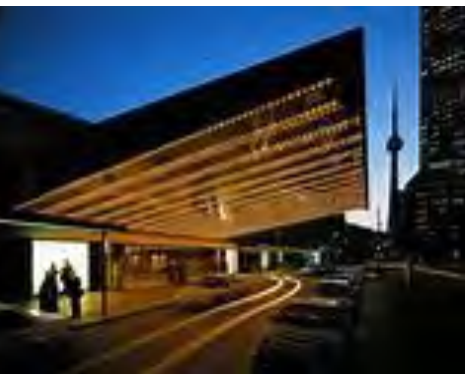
ACO Award Nominee Meridian Hall restoration, ERA Architects
